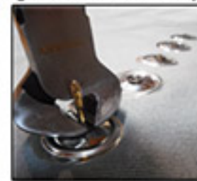
Cut off excess nail shank
