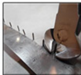
Using a thin object for spacing, cut down exposed nail shank
